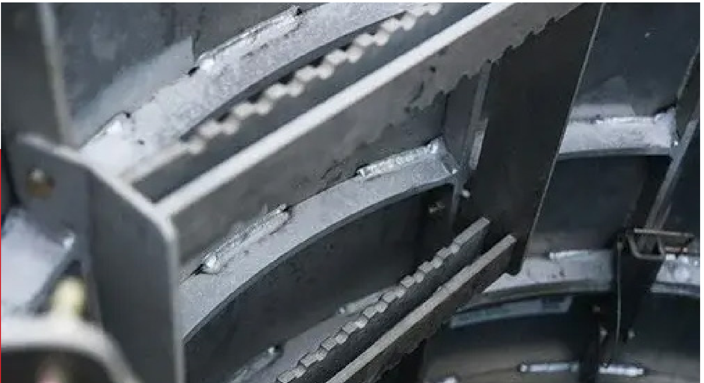
Inside an installed EasyDig cage. The ladder is built into the panel.
