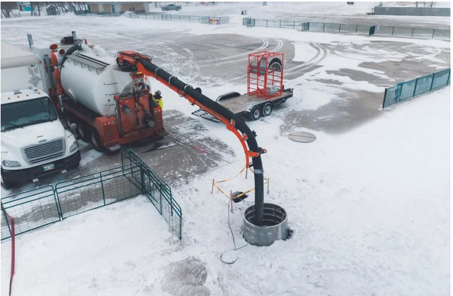
Aerial view of an EasyDig installation paired with a hydrovac truck. Photo courtesy of EasyTech Infrastructure Group.
